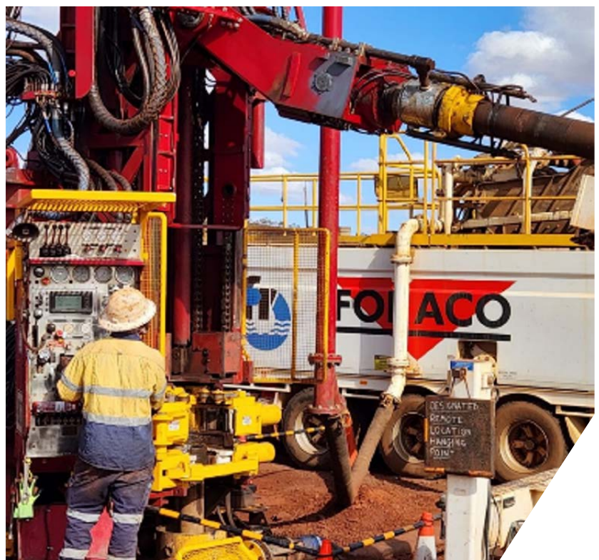
Driller on traditional rig control panel drilling 17.5" Large Diameter Flooded Reverse (LDFR) water wells.
